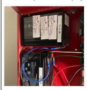
FAILURE REASON: Check charger. Set of 12v 7.5ah batteries failed load test at 80%. Need replacement.
