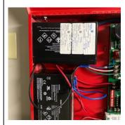
2nd Floor | Electrical Rm in hall by suite 240 BPS#6 | Battery | — FUNCTIONAL FAILURE | DEFICIENCY IMAGES APPENDIX 1.5
