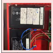
FAILURE REASON: Set of 12v 7.5ah batteries failed load test at 80%. Need replacement.
